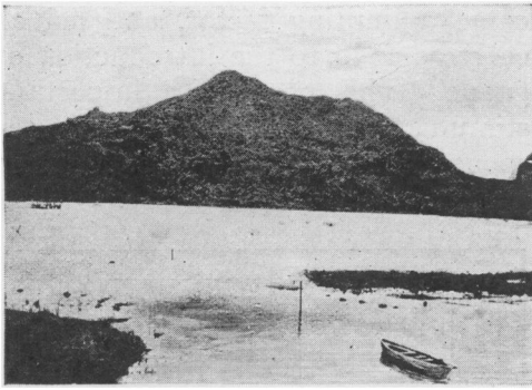
FIGURE 7.—La Ferme Reservoir in the dry West of Mauritius is formed by diverting the surplus water of two streams and irrigates over 3,000 acres. (Courtesy of "Empire Production.")
